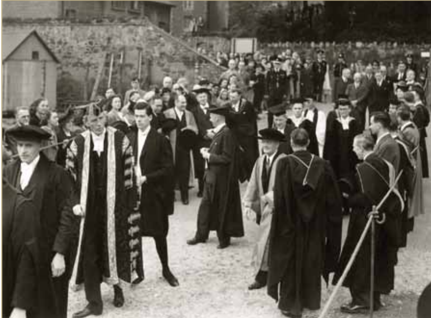
21 April 1949: Fellows of the College are presented to the Founder at the ceremony of laying the foundation stone for Nuffield College. Lord Nuffield is towards the centre of the picture in a pale gown, walking towards Lord Halifax, Chancellor of the University (to the left of the picture in the heavily embellished gown).
