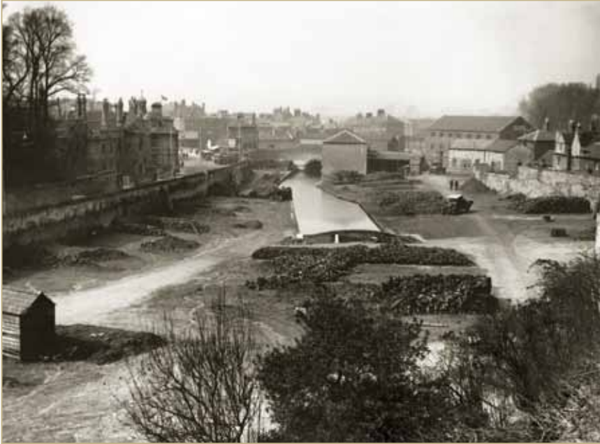
The college site as a coal wharf just prior to the start of building work.
